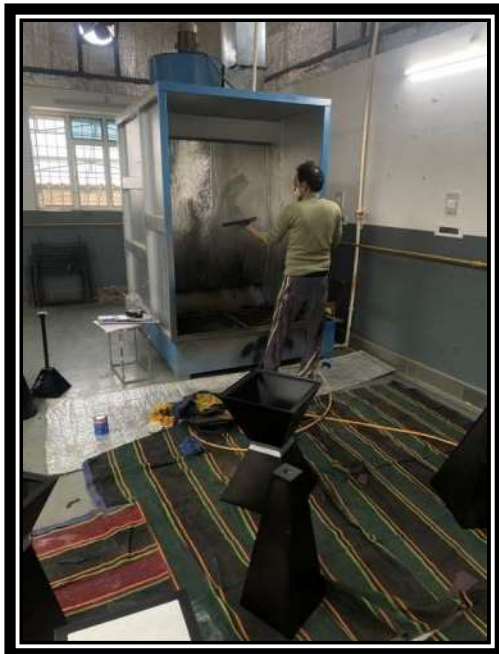
PAINT / LACQUER ROOM
