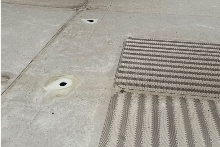
Sealant applied over holes
